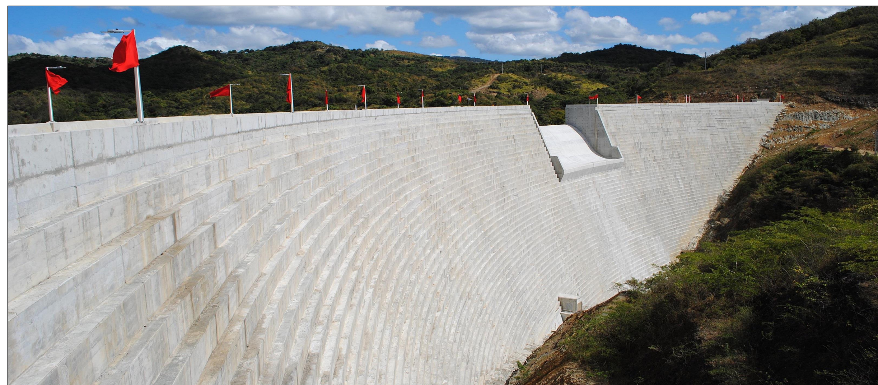
Figure 1. Aerial view of the Portugues Dam
