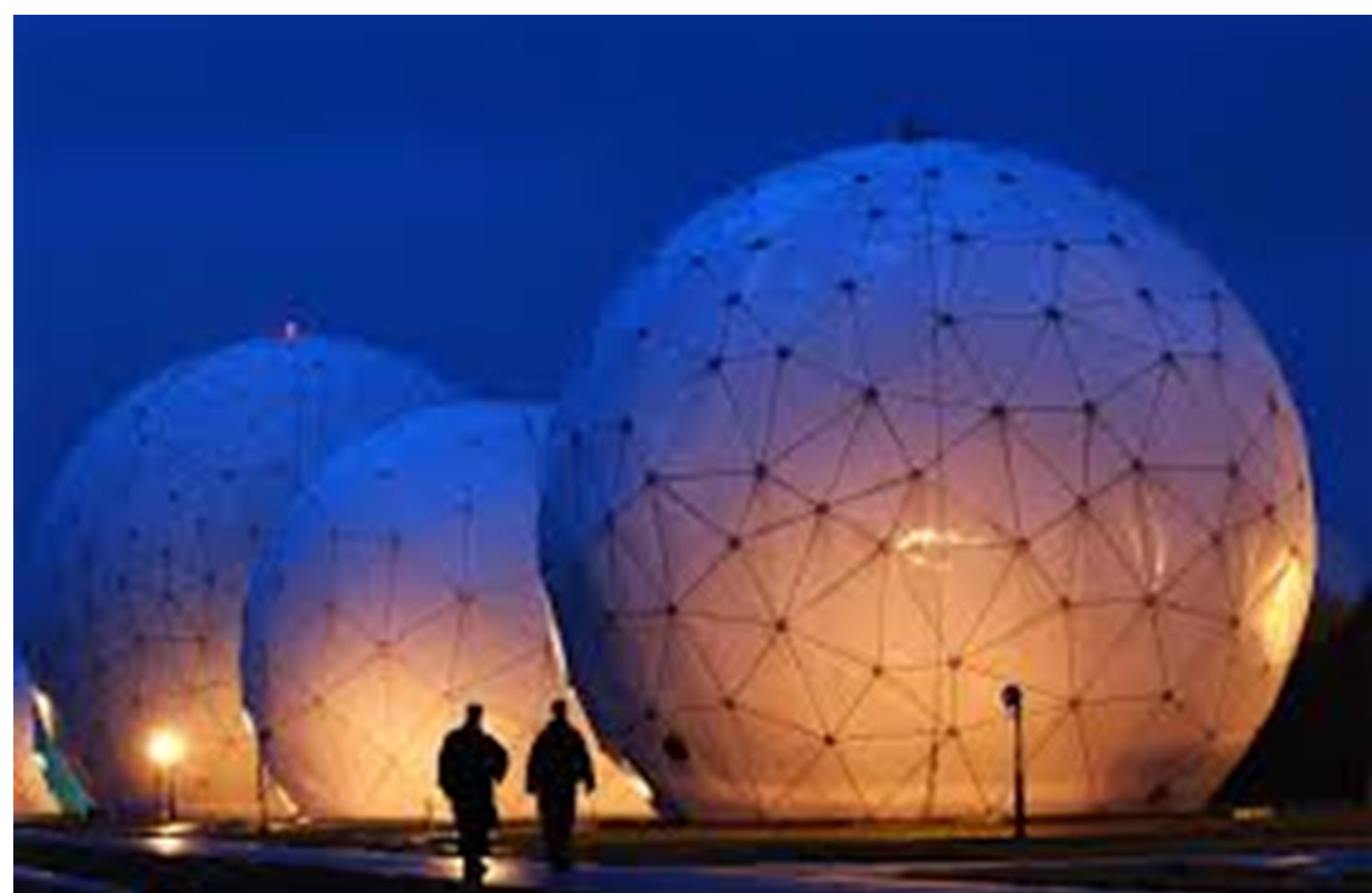
Figure 1. Ground based spherical radome. (src: Wikipedia)
